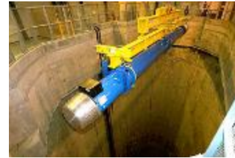
1st LHC cryo-magnet lowering
