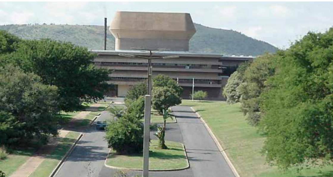
Figure 8: Paramic view of the 20 MW SAFARI-1 research reactor building.
